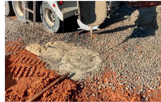
Provide washout containers to avoid discharging concrete onto the ground.
