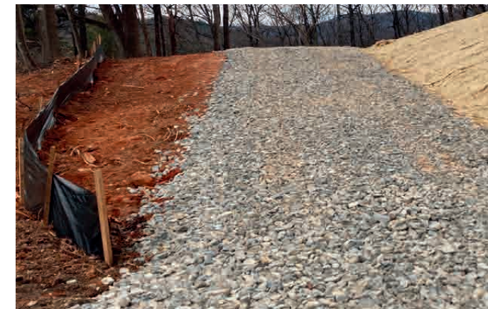
Use VDOT #1 stone over geotextile fabric for construction entrances to prevent sediment tracking onto paved or public roads.
