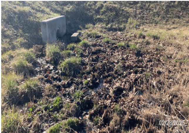
Remove accumulated sediment below the southeast inlet pipe and reinstall outlet protection.
