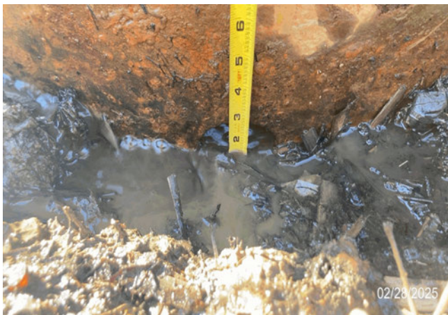
Remove accumulated sediment from around the outlet orifices.
