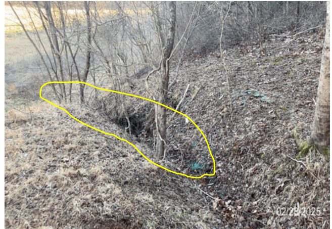
Remove trees and repair erosion within the southwest inflow channel.
