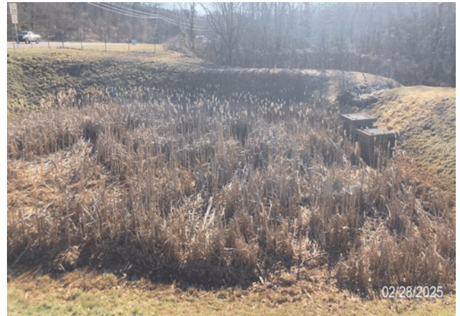
Remove accumulated sediment and cattails. Grade the basin to restore design dimensions. Stabilize all bare areas once grading is complete.
