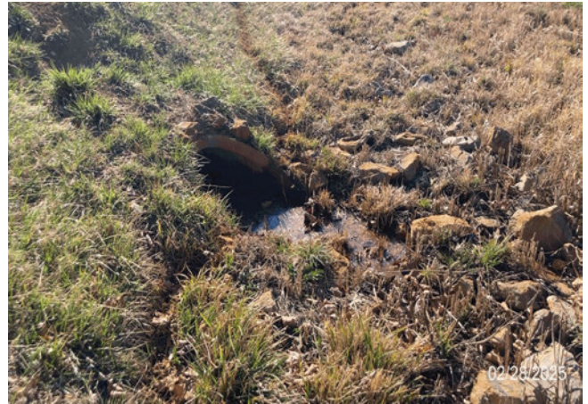
Remove accumulated sediment below northeast inlet pipe and reinstall outlet protection.
