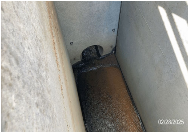
Install a restrictor plate as per the approved plan.
