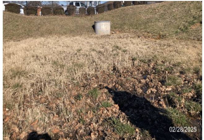
Remove accumulated sediment and grade to ensure positive drainage. Stabilize all bare areas once grading is complete.
