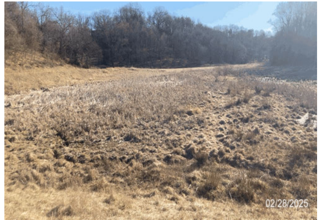
Remove accumulated sediment, cattails, and saplings. Grade the basin to restore design dimensions and ensure positive drainage. Stabilize all bare areas once grading is complete.
