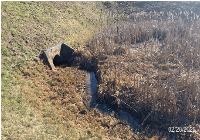
Remove accumulated sediment from within and below the inlet pipe. Reinstall outlet protection once the sediment is removed.
